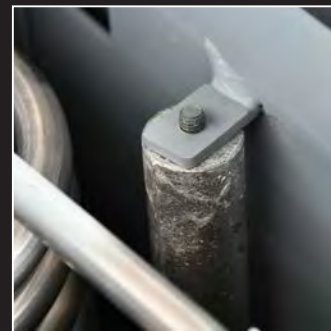
Magnesium sacrificial anode for added protection of the boiler
